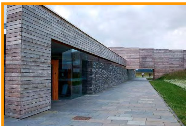
Scotlarch cladding (Russwood of Newtonmore) - trials of alternative finishes at the sawmill and as installed on NTS Culloden Battlefield Centre
