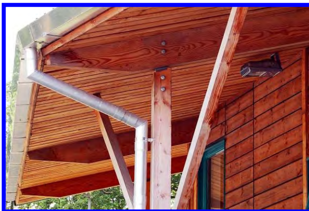
Scottish-grown Douglas fir roof-trusses in new Forestry Commission district offices at Huntly (below) and Smithton, Inverness (above)
