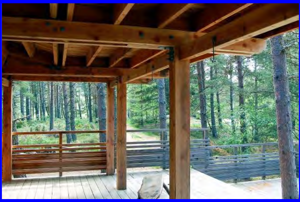
Douglas fir used for simple post-and-beam construction in Scotland - community forest cabin (above)/ David Douglas Pavilion, Scone
