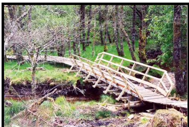
Uses of western hemlock - treated landscape sleepers and mountain-bike Northshore boards
