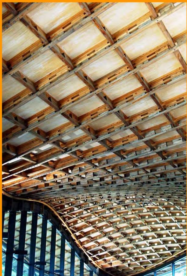
Larch gridshell roof - Savill Building, Windsor
