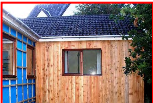
Local use of rustic western red cedar cladding in Highland Scotland - an alternative to larch
