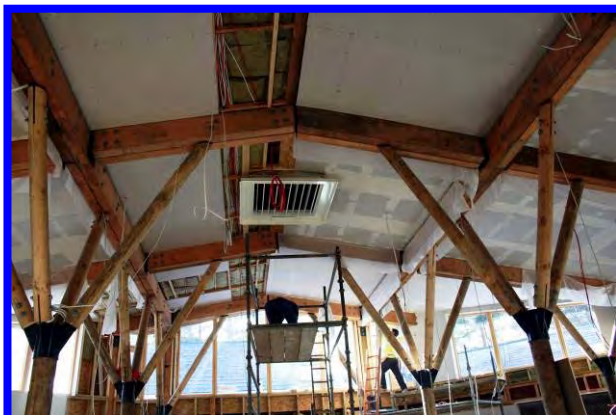
Scottish-grown Douglas fir roof-trusses in new Forestry Commission district offices at Huntly (below) and Smithton, Inverness (above)
