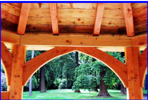
Douglas fir used for simple post-and-beam construction in Scotland - community forest cabin (above)/ David Douglas Pavilion, Scone
