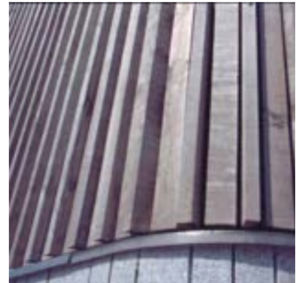
Figure 9.9.7 Detail - metal drip protecting the masonry below from tannin run-off Photo: P Ross
