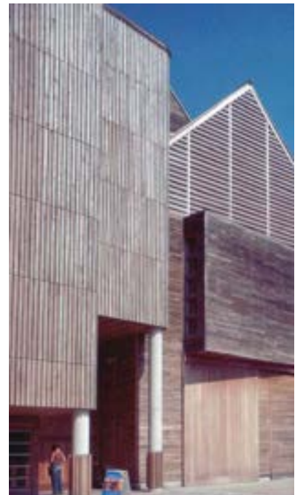
Figure 9.9.2 Intermix of cladding details Photo: P Ross
