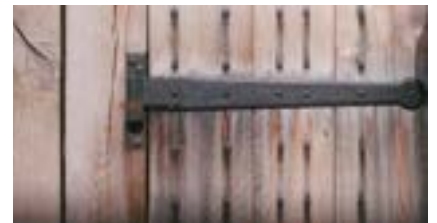
Figure 9.1.10 Staining from the iron nails in the door Photo: P Ross
