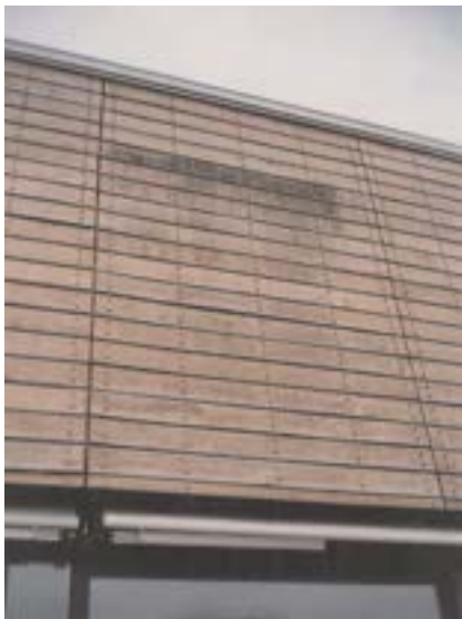
Figure 4.12 Tannin exudation on European oak cladding boards
