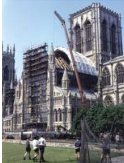
Figure 9.5.7 Lifting four complete trusses in one day required a crane with a lifting capacity of four tonnes at a twenty metre radius, but this was an economic alternative to dismantling and re-erection Photo: P Ross
