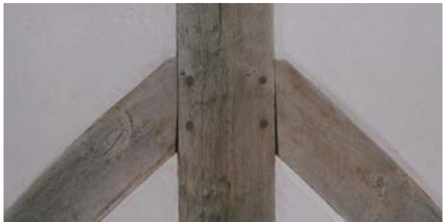
Figure 9.1.7 The typical wedge-shaped drying movement at the ends of the wind braces Photo: P Ross
