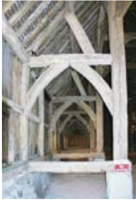
Figure 2.1 Aisle at Harmonsworth Barn, Middlesex. Photo C J Mettem
