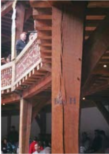
Figure 9.1.4 The major fissure in one of the ground floor posts Photo: P Ross
