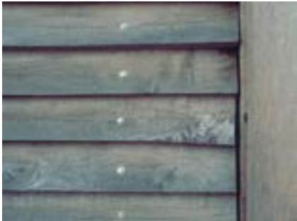
Figure 9.9.5 Detail B Lapped boarding. Small in-plane drying movements can be seen, together with a large knot in the third plank down Photo: P Ross
