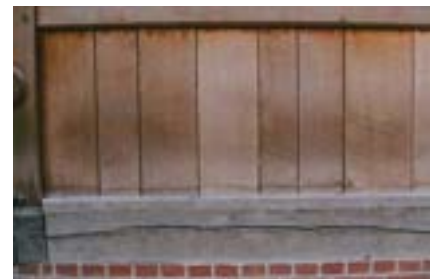
Figure 9.1.11 The sill beam, showing water marking and darkening on the planking above where 'groundlings' squat on the beam Photo: P Ross
