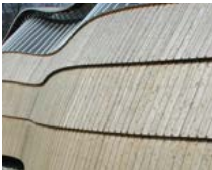
Figure 9.8.7 At the entrance the shell connects to a European larch glulam arch Photo: Buro Happold / Weald and Downland Museum
