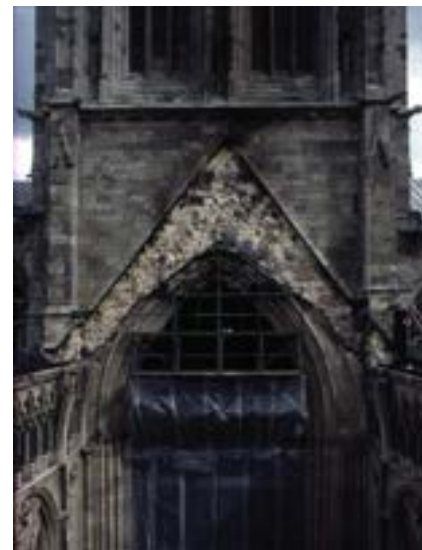
Figure 9.5.2 The south face of the central tower immediately after the fire, showing the dripstone which sets the line of the roof, and below it, the line of the vault Photo: P Ross
