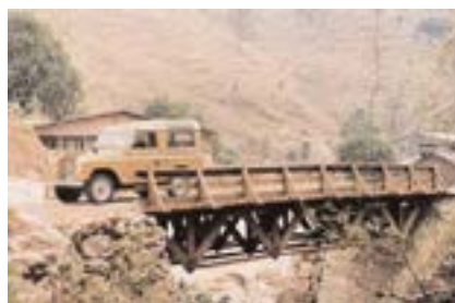
Figure 8.22 Modern system-built light vehicular bridge, widely used in several world regions. Suitable for incorporation of strength graded air-dried European oak Photos: C J Mettem
