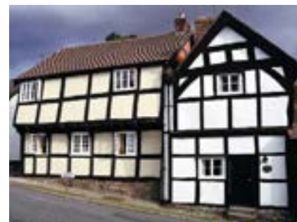
Figure 8.2 The technique of building oak frames using sill beams mounted on stone or brick was developed quite early, because earth-fast posts rotted quickly. A horizontal sill beam resting on a low stone wall resists ground water because moisture absorption across the grain is much more limited than through the end grain. In conjunction with modern damp proof courses and flashings, this is still best practice (Weobley, Hereford and Worcester)
