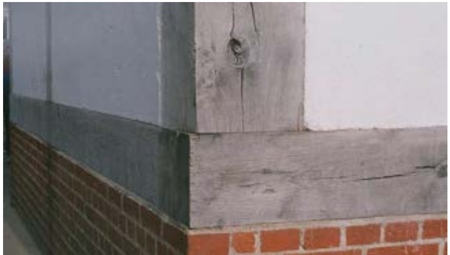
Figure 9.1.6 Slight twist at the base of one of the posts in the north-east tower Photo: P Ross
