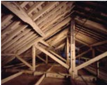
Figure 2.8 King post truss. Roof of Trinity College, Cambridge. Photo: Jewell Harrison
