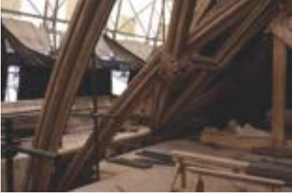
Figure 9.5.11 The assembly of the vault, with ribs tenoned into bosses (also made from oak strips, brick bonded to keep the grain in one direction out of consideration for the carvers)
