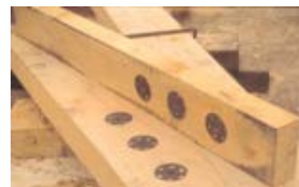
Figure 9.5.5 The scissor straps before assembly, showing the double shear connectors which will eventually be back-to-back on the same bolt. The connectors move with the timber they are set into, and do not lose strength if the timbers distort while drying Photo: P Ross
