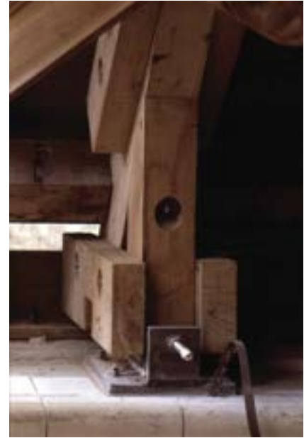
Figure 9.5.8 The east truss legs rested on a sliding bearing and were restrained by a threaded rod engaging with the upstand arm of a cleat bolted to the masonry. As the load of the roof boards and lead covering were applied, the leg restraint was gradually released by unscrewing the nuts in sequence, a quarter-turn at a time. Most of the out-thrust was dissipated, leaving the scissors acting as true trusses Photo: P Ross
