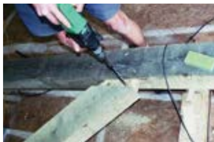
Figure 5.34 Draw boring a tenon in a raking brace
