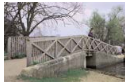
Figure 8.17 A typical oak footbridge of modest scale on the Thames towpath, at Marlow, Buckinghamshire. The parapet design reflects a famous nineteenth century suspension bridge crossing the river nearby Photo: C J Mettem
