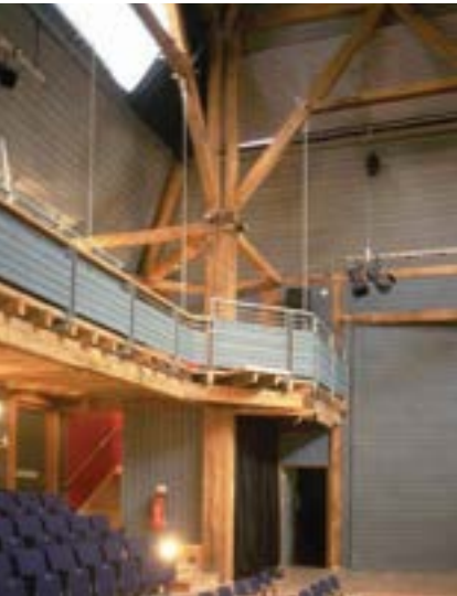
Figure 9.6.3 Balcony support Photo: P Ross
