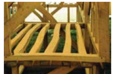
Figure 6.11 Floor joists, traditionally hand sawn only on what became the upper and lower faces, placed “flatwise,” and hence providing a level floor
