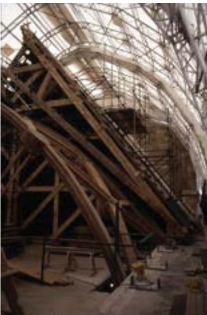
Figure 9.5.12 The relationship between the vault and the trusses
