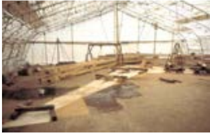
Figure 9.5.6 The temporary covered workshop set up on the north side of the nave. The plywood floor is painted white and the truss profiles drawn on it. In the photograph, two trusses have been fabricated and stacked to one side by lifting with shear legs Photo: P Ross
