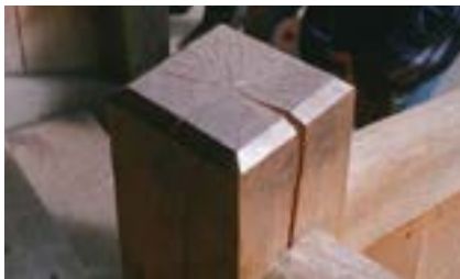
Figure 9.1.5 A newel post with boxed heart showing radial fissures. The handrails, being quarter-sawn and excluding the heart, have few fissures. The polish on the top of the post is entirely due to hand contact Photo: P Ross
