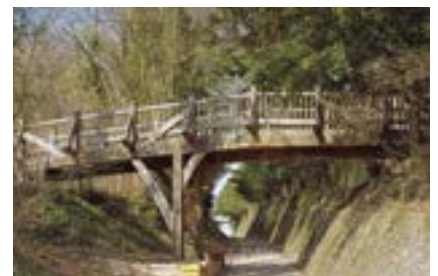
9.11 Polesden Lacey bridge
