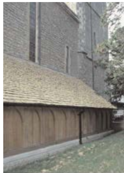
Figure 8.10 Protecting key elements. The Cloister Pentice, Dorchester Abbey. A new-build in green oak, exposed externally and well designed with regards to protection. There is an eaves overhang; the timber is elevated on a masonry sill well above the splash zone, and there is an effective rainwater drainage system Photo: P Ross
