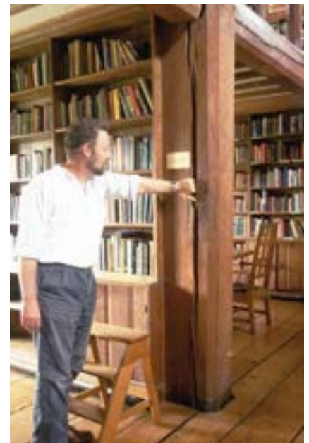
Figure 5.7 Significant fissure in a post in Bedales School library, built in 1921 Photo: P Ross
