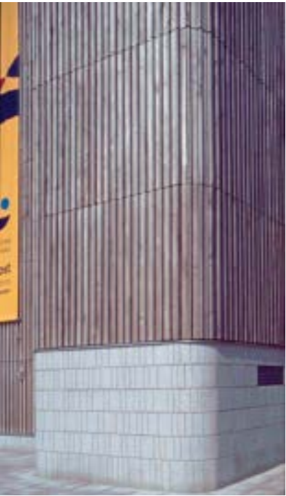
Figure 9.9.4 Alternate batten detail used on the curved wall surrounding the main entrance Photo: P Ross
