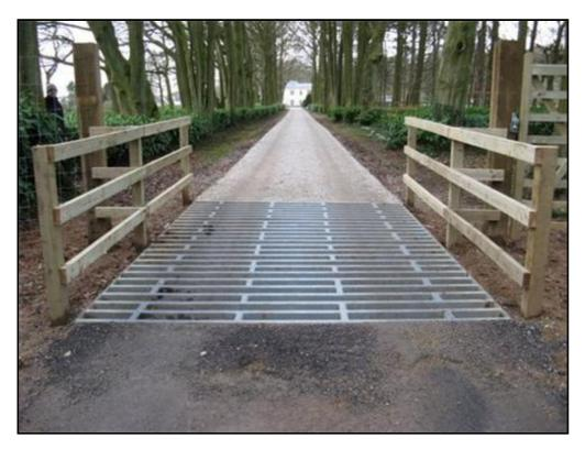
The grid will be made to a standard highway grid specification with a jump width of 15ft 3ins (as in photo above) and it will be manfactured to fit the road it is going on. It will have a wooden pedestrian gate (similar to photo below) designed with best practice in mind on the side nearest the bridge
